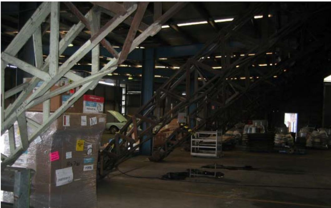
Figure 5: Interior of Hangar No. 7 showing timber box frame trusses
